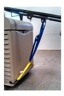
Once the front lift bar is securely in place, insert yellow strap in the two rear shipping holes of the generator. Install one end of the blue strap to the yellow strap and the other end to the hook at the bottom of the handle.
