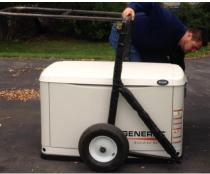
Insert crossbar into middle (Kohler) generator shipping holes. Install cotter pins to secure bar.
